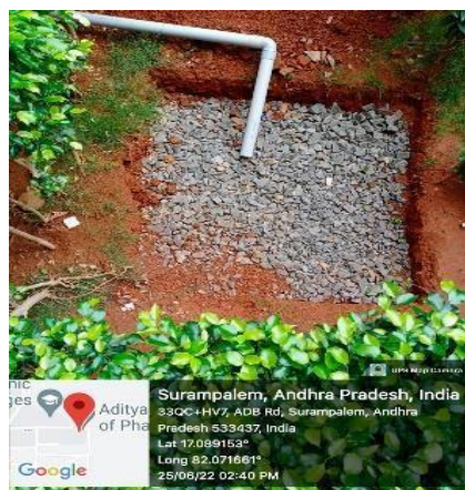
Construction of Recharge Pits
