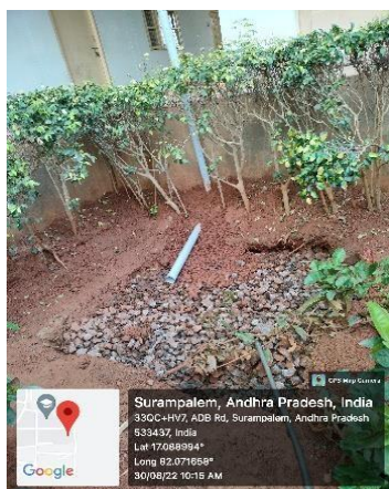
Construction of Recharge Pits
