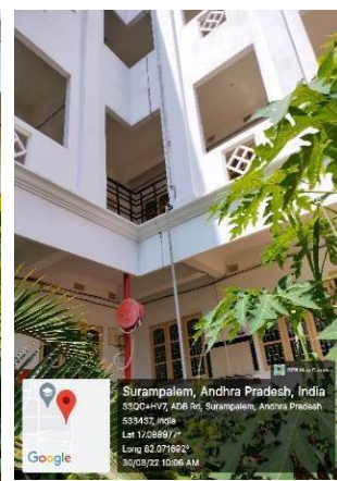
Pipe fitting from terrace top connected to the recharge pit
