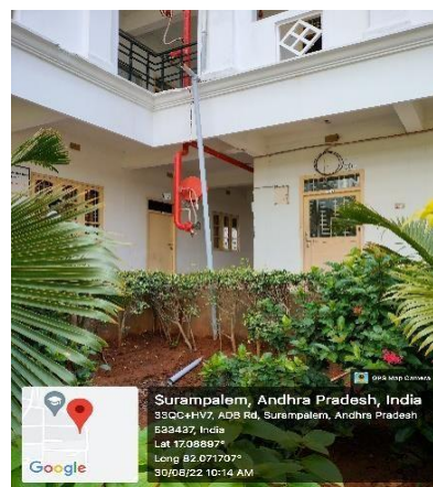
Pipe fitting from terrace top connected to the recharge pit
